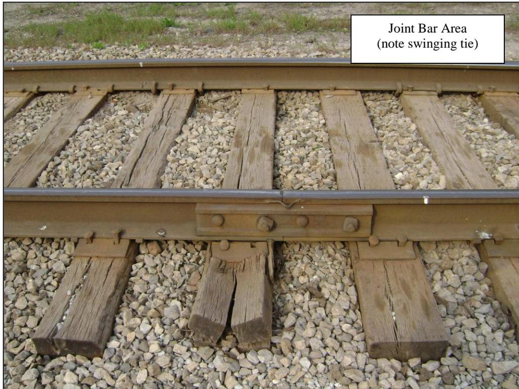
welded rail (CWR), the best method to improve ride quality is through elimination of joints. Costs are estimated in the next section and detailed in Appendix A.
